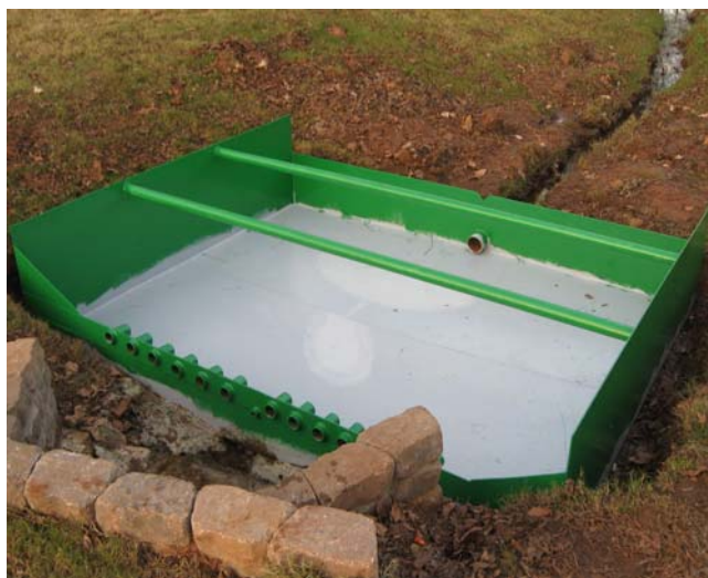
Figure 1. The uncompleted phosphorus removal structure shown during construction.
