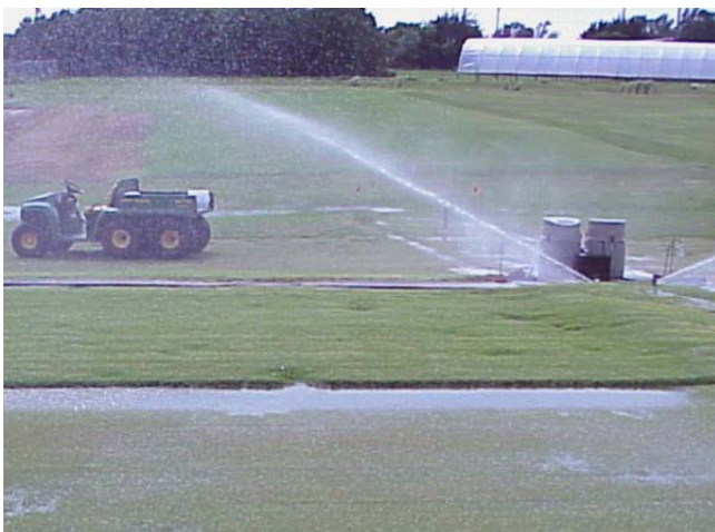
The irrigation system provided precipitation at two inches per hour resulting in applications of 905 gallons per acre per minute.
