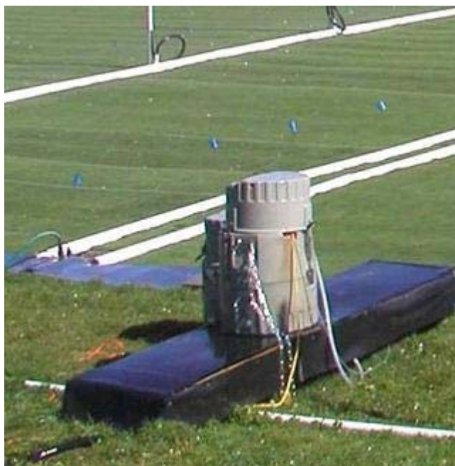
Automated samplers and flow meters recorded volumes, measured flow rates and collected runoff samples.
