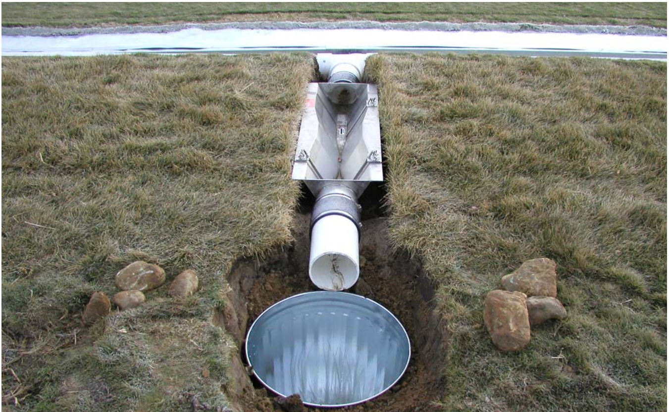
Runoff gutter and trapezoidal flume for collection of runoff.
