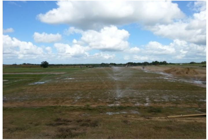
Figure 4. Initial establishment of the sandcapping research site. The subsoil was graded to provide a uniform 2% turtleback up through the center of the site facilitating subsoil drainage of excess water to the
