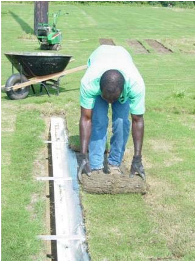
**Figure 2.** Installation of runoff diverter and collection trough.
