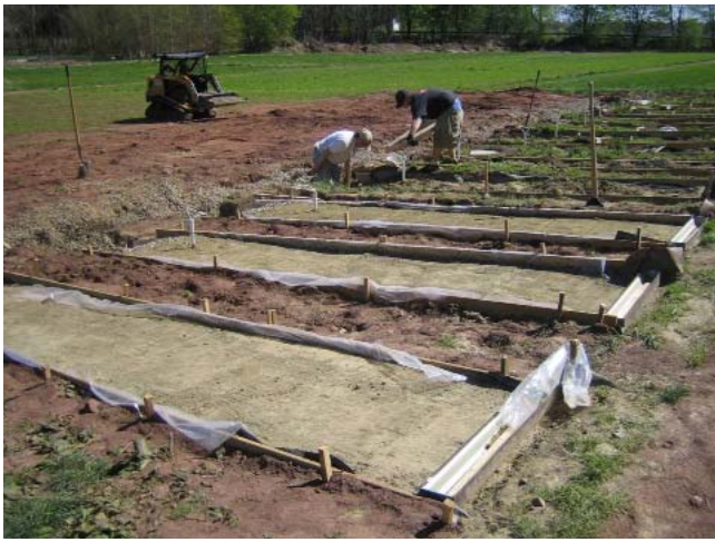
Figure 7. Plastic liners were installed over the edging of each pre-planted VFS and the soil was graded to 5% slope.
