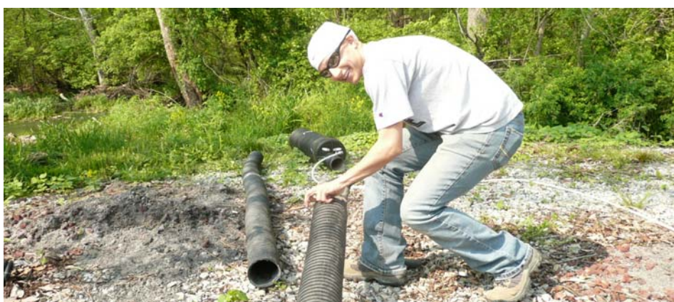
A subsurface pipe with flow control structure was installed to route irrigation reservoir water at the western edge of the course through two corrugated black tiles.
