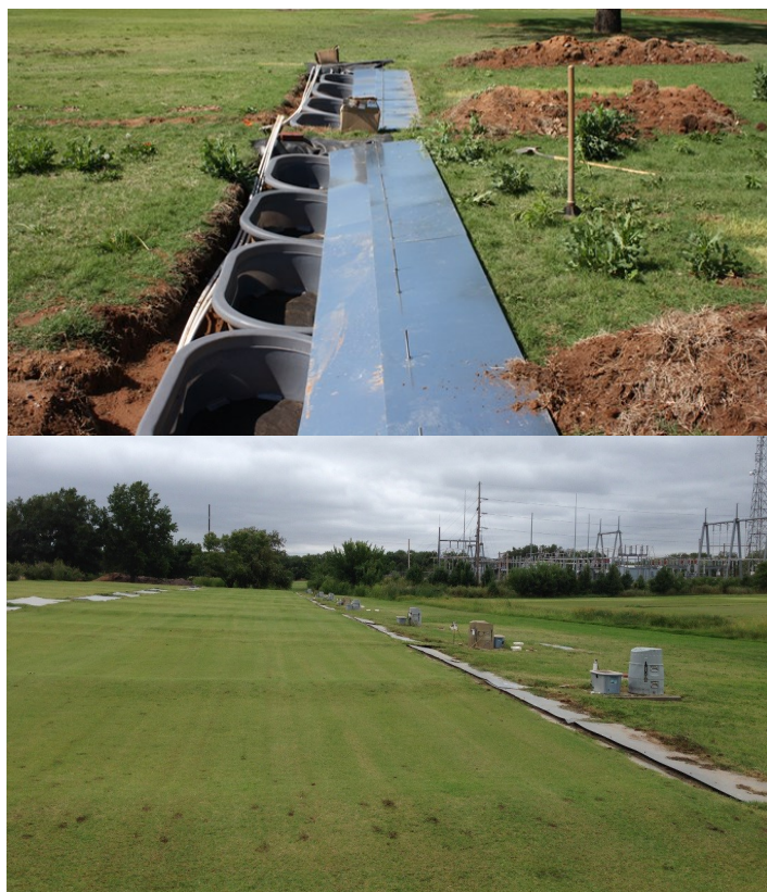
Figure 1. Construction of the slag interception trenches on the runoff plots located at the Botanical Gardens at Oklahoma State University (Top photo). Tubs were filled with steel slag ( >6.35 mm) to allow runoff (perpendicular to trench) to flow into the phosphorus sorption material before draining into plastic pipe. ISCO samplers collected drainage water to determine the amount of phosphorus present.
